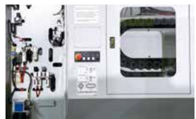
F. Centralized Configuration Lubrication and pneumatic panel easy to maintenance.
